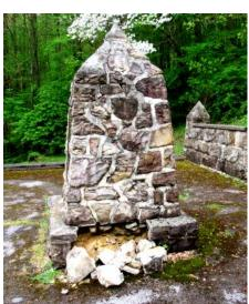
damaged, with some loose stones knocked out near the base and cracks developing between all of the stones. Also, there has never been a sign at the end of the road leading from Route
